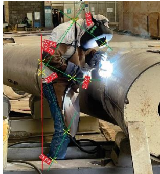
Figure 1. Work Posture for Assembling Metal Duct Components of Worker 1
