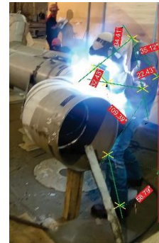
Figure 4. Work Posture for Assembling Metal Duct Components of Worker 4
