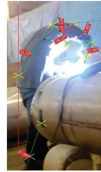
Figure 3. Work Posture for Assembling Metal Duct Components of Worker 3
