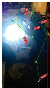
Figure 2. Work Posture for Assembling Metal Duct Components of Worker 2
