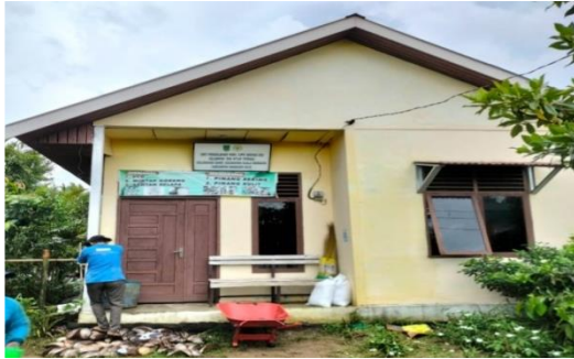
Figure 1 VCO Production Building
